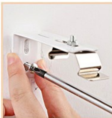
05. Fix the installation code on the wall
